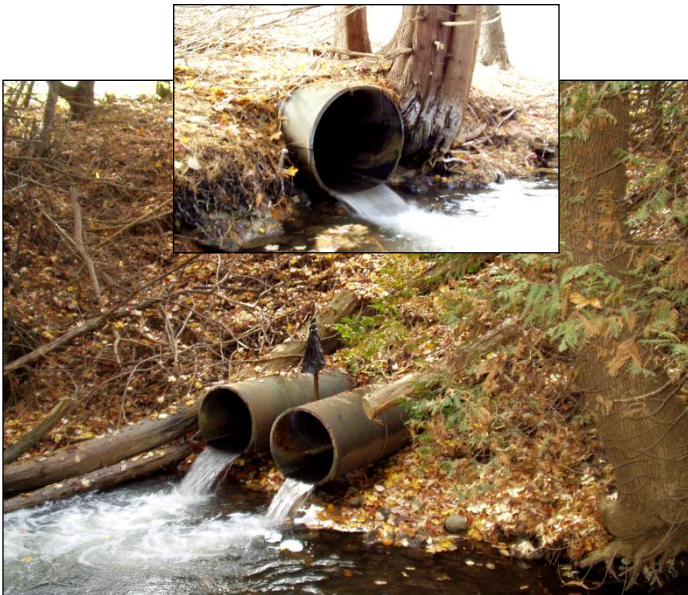
Boardman River (Ottawa River) tributaries crossed by the GLC Railroad and Cass Rd. in Grand Traverse County; bottomless structures will be designed to facilitate fish passage.
