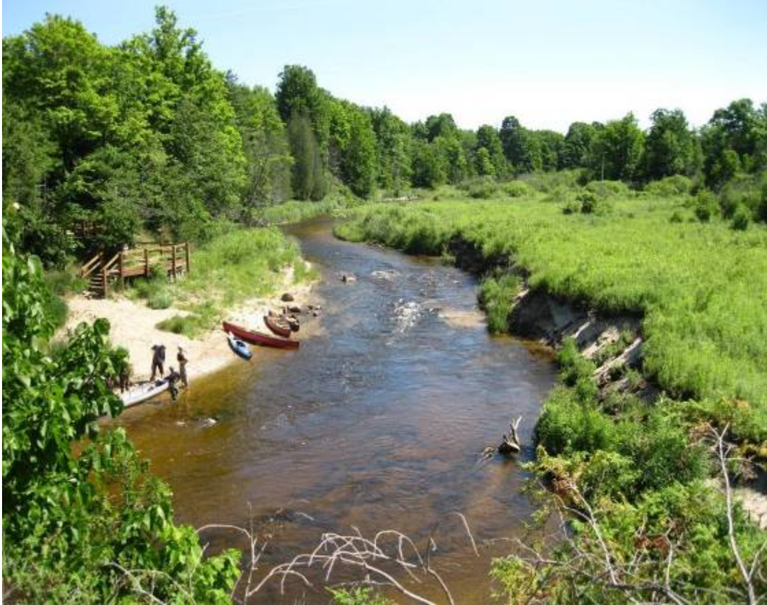
Figure 10. Former Boardman Pond and Resulting Channel Cut through Material Deposited Upstream of the Dam
